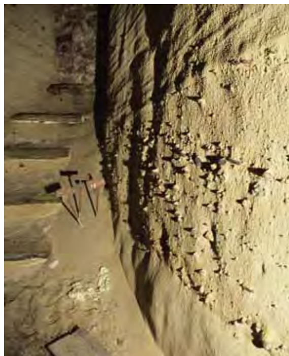
In Thomas Herbert's herbarium cave, projecting pebbles and a bank of fallen sand along the foot of a wall indicate the loss of the sandstone by weathering.
