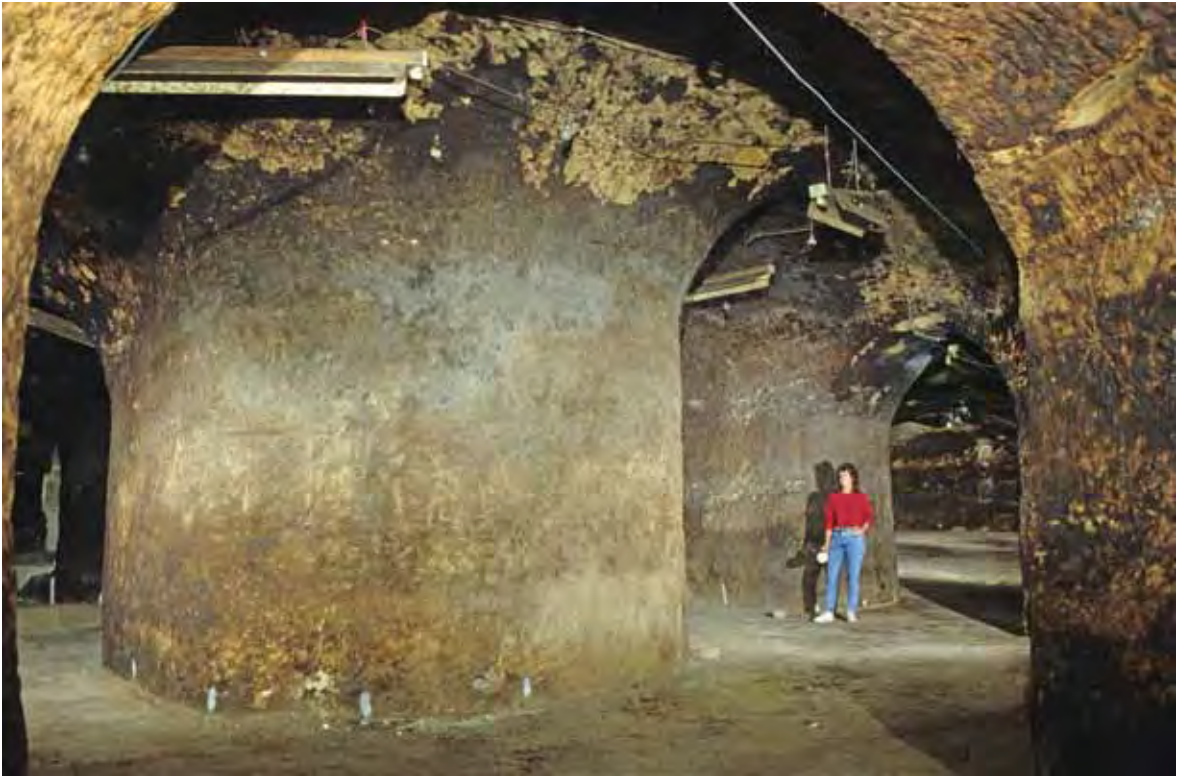
Massive sandstone columns between the spacious caves that were excavated to become the cold store for Burton's, the Victorian purveyors of fine foods
