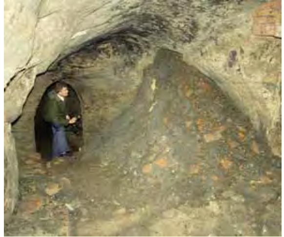
The pile of debris that landed in the lower of the Black's Head caves when the saturated sandstone and the soil fill collapsed in the malt kiln cave above.
