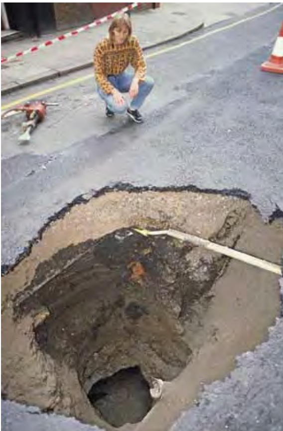
The crown hole collapse in Stanford Street; most of the open hole is in soil and fill, but rock is just visible around the dark hole breaching the cave roof.
