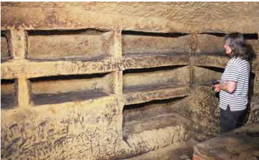
Shelves cut into the sandstone walls of one of the group of storage caves that survives beneath Gawthorne House on Low Pavement. Though so many caves were mainly used for storage, these are the only rock-cut shelves now known..
