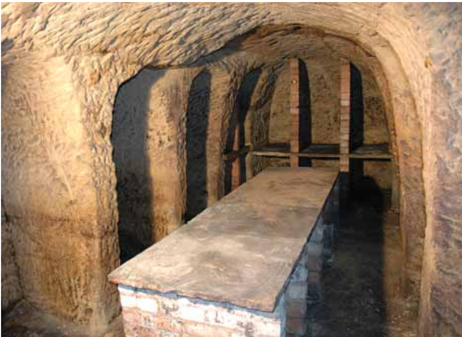
A fine small cave recently found under a house on Forest Road. The sandstone partitions between the alcoves along the walls are typical of a wine vault, and the large central table has a top of natural flagstone standing on columns of brick.
